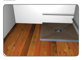
Paint acrylic primer onto the edges of the shower tray and onto adjoining walls, covering at least 50mm of tray and wall. Allow to dry. From a roll of sealing tape cut to suit the width of the shower tray and the length of the shower tray. Temporarily place a waterproofing internal corner into position and mark around it with a pencil. Once marked it can be removed. This is to show where you need to apply Tanking Solution. Repeat for any other corners.
