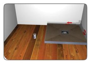
Using the Tanking Solution and a paintbrush, apply a thin layer of Tanking Solution to the Internal Corners of the shower tray, slightly bigger than the pencil line marked earlier. Place the waterproofing Internal Corners into the internal corners of the shower tray and push firmly into the Tanking Solution. Apply a further thin layer of Tanking Solution over the edges of the waterproofing Internal Corners.
